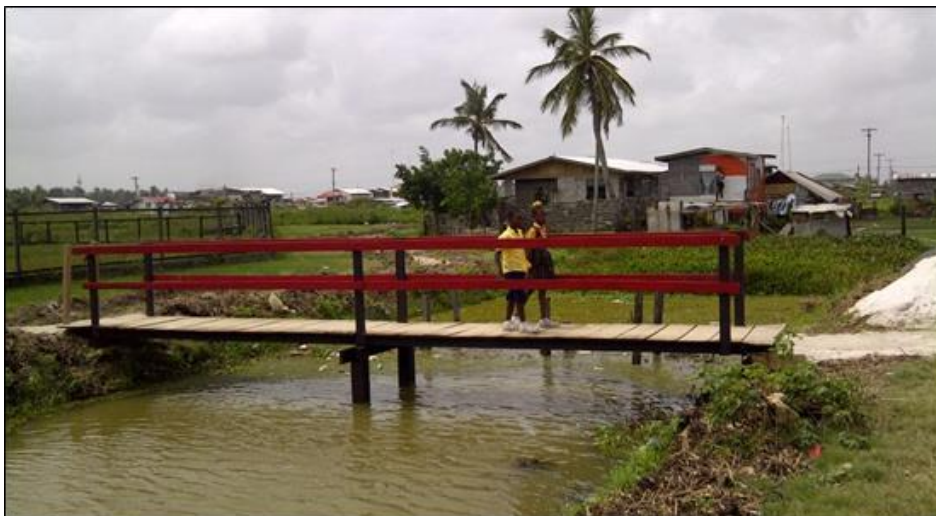
Bridging Gaps: The Golden Grove/Nabaclis/Haslington Group (Region IV) obtained funding from the READ project's Productive & Social Investment Fund for dam rehabilitation and a new bridge to improve farmers' productivity, enhance opportunity for enterprises and improve living conditions for women, school children and the elderly in the community.
