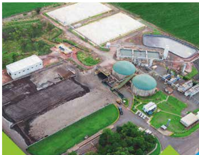
FIGURE 50. Geo Elétrica Tamboara biogas plant
